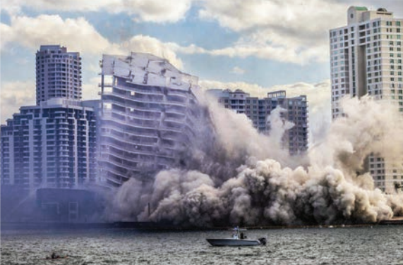
Mandarin Oriental Hotel Demolished on April 12, 2026 2026
